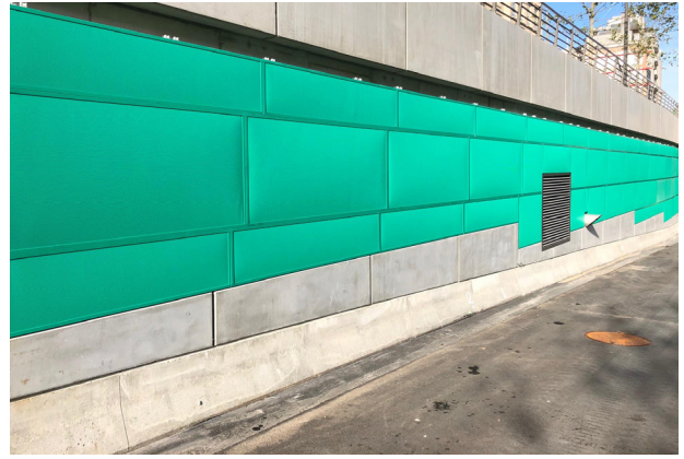
Absorberende tunnelwandbekleding, Brabotunnel, Antwerpen
